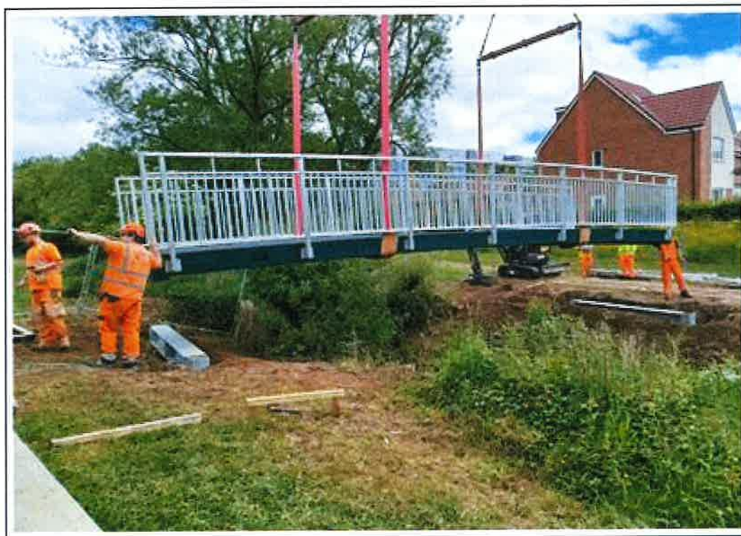
Figure 1-2 - Example Bridge Construction
